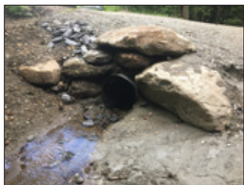
New culvert at the Mill Trail
